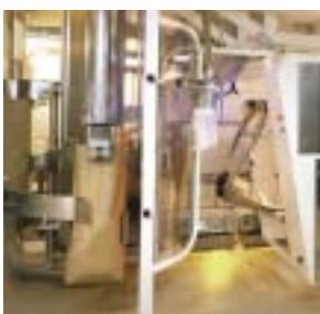
Automatic Avalon carousel bagging-off equipment
