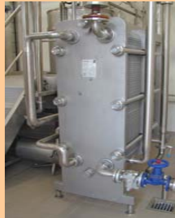
Plate heat exchanger
