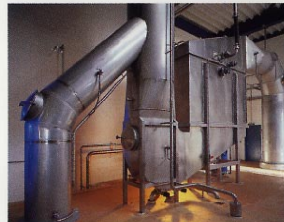
Air exhaust ducting and heat recuperation unit equipped with CIP nozzles.
