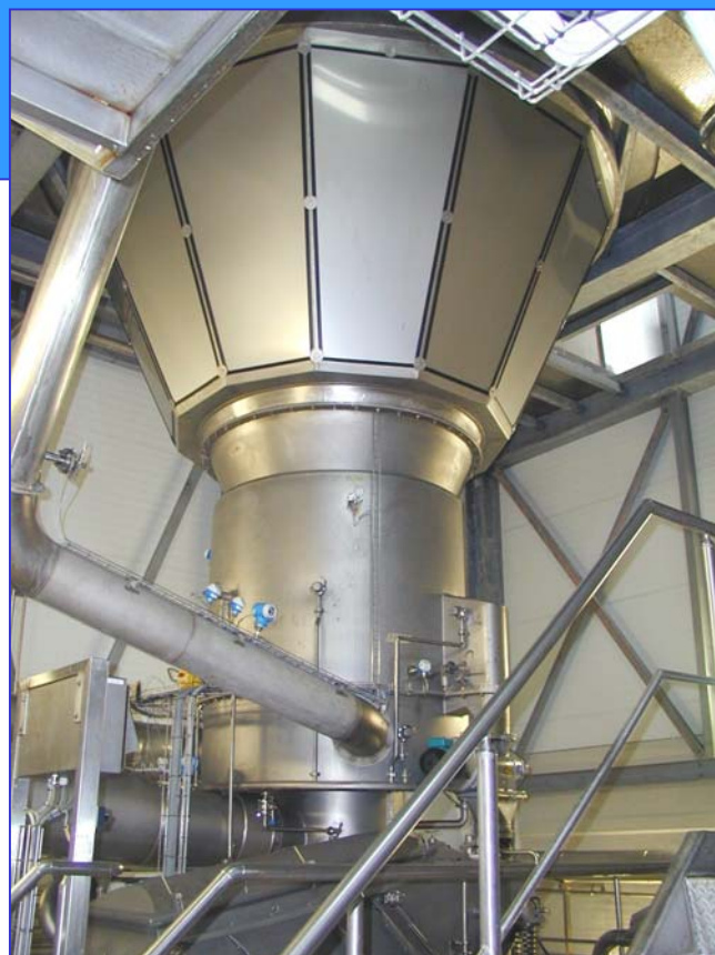
The Integrated Filter Dryer - IFD™ installed at Arla Foods' factory, Videbæk, Denmark. Photo shows lower part of drying chamber and the integrated fluid bed.
